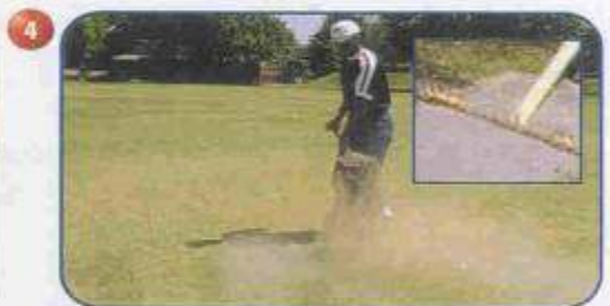
Spread a good quality top soil over demarcated area and rake to fill any indentations.
