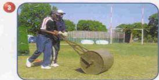
Roll area with medium weight roller to remove all bumps.
