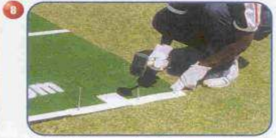
Ensure pitch is in correct position, then, using either 4" (10 cm) or 6" (15 cm) nails, secure pitch by hammering nails into holes in edging strip.
